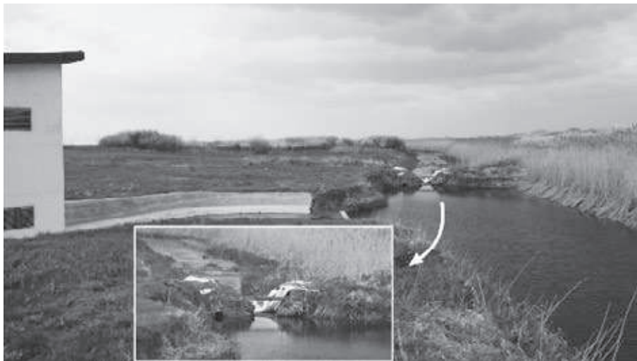
Pumping station - Plot Aranca Photo: Judith Bouniol - Dudeștii Vechi - April 2012
